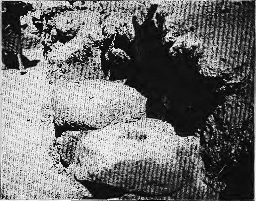
FIG. 71.—CUP FOR RECEIVING THE HORN OF A DOOR
